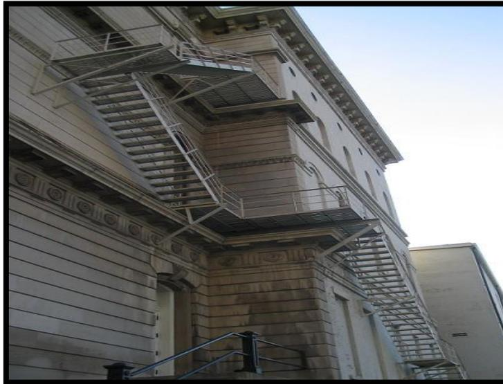
*Figure 2.109: fire escape located external to a building*
