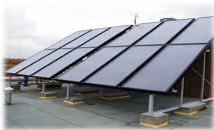
*Figure 2.27: flat plate collector*
