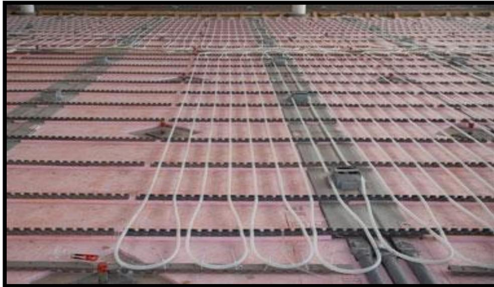
Figure 2.73 under ground: radiant cooling system
