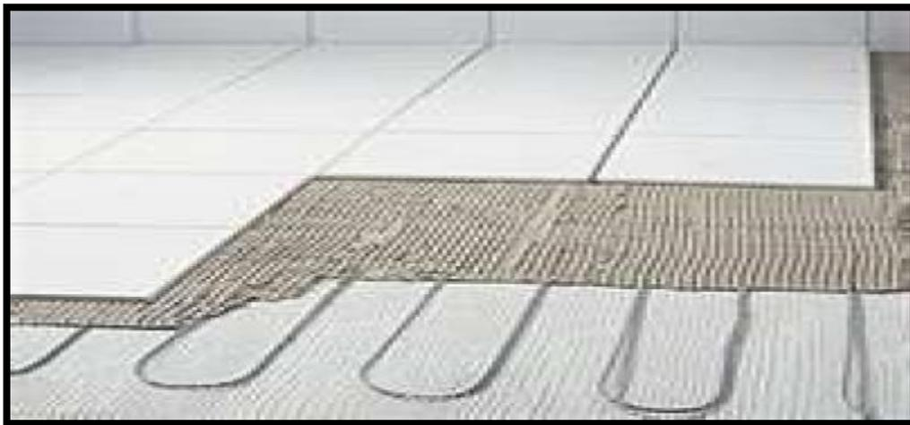
*Figure 2.68: radiant floor heating*
