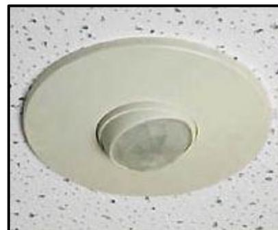
**Fig. 3.9.4** Example of a ceiling-mounted occupancy sensor.
